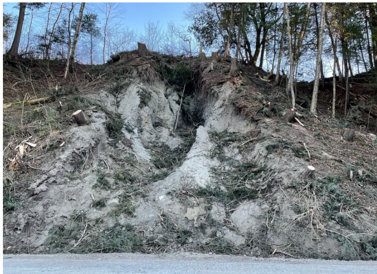
Figure 1. Slope looking South, gully erosion characteristics present in upper half of slope
